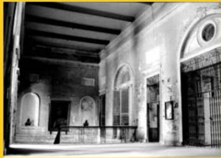
The Town Hall – upper landing before restoration
